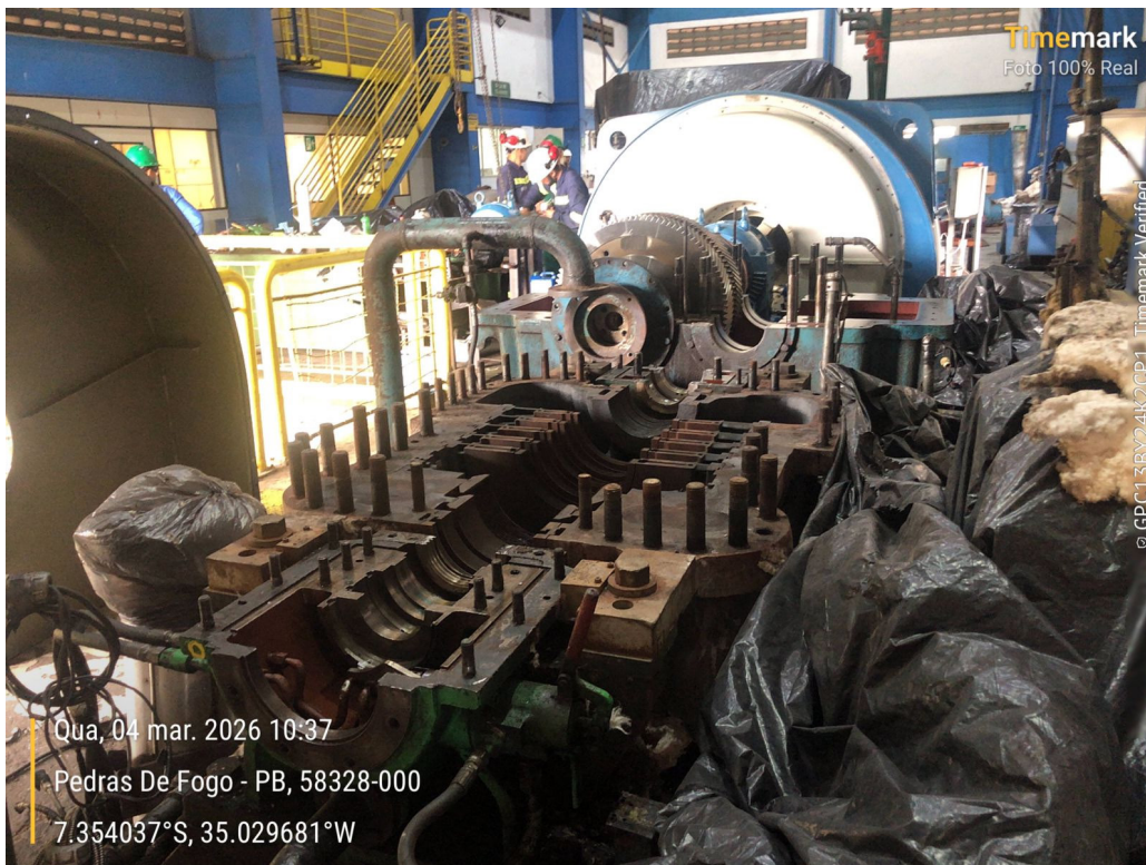
Generator UG8 - Turbine under preventive maintenance
