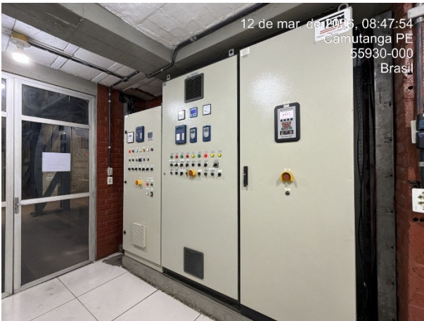
Turbine Control Panels
