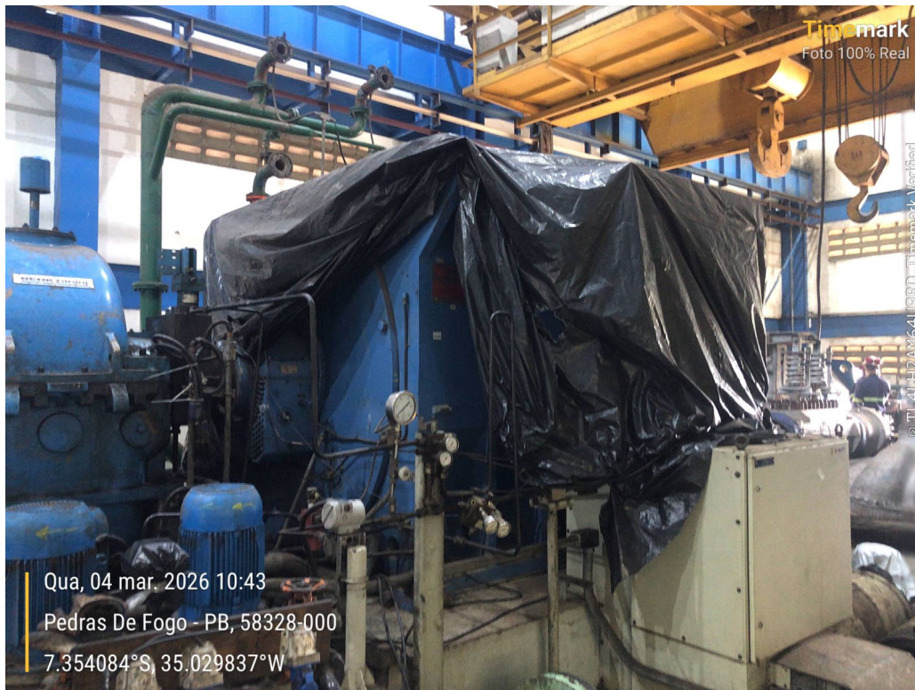
Generator UG9 under preventive maintenance
