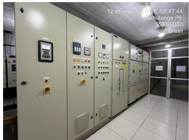
Turbine Control Panels
